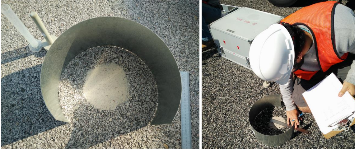
Figure 2-4 (a) Sand Patch test equipment, and (b) field data collection
